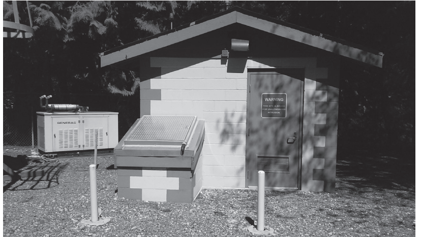
Braunwood Pump House
