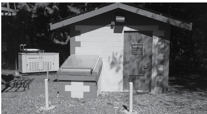
Braunwood Pump House
